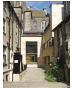
Top , the south or New Combination Room end of Hostel Yard facing, centre , the now demolished north end. Constructed, in 1929, of similar materials, but designed in different styles, the two ends of the Yard complemented each other and took their cue from their context.
