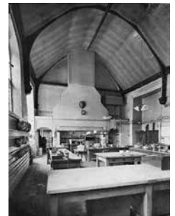
The former medieval Hall, shown here in use as the kitchen, before a mezzanine was inserted in 1948
