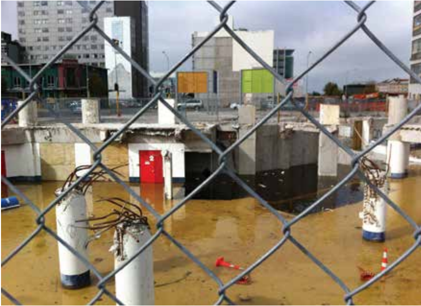
Basement of a deconstructed building in city centre, Christchurch
