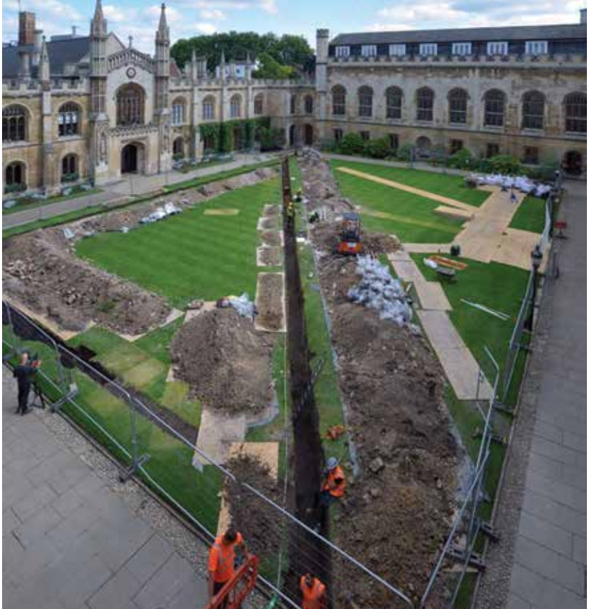
New Court, during the excavations for the power cables
